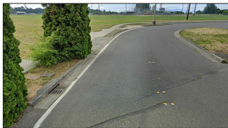
VIEW LOOKING SOUTH WEST
