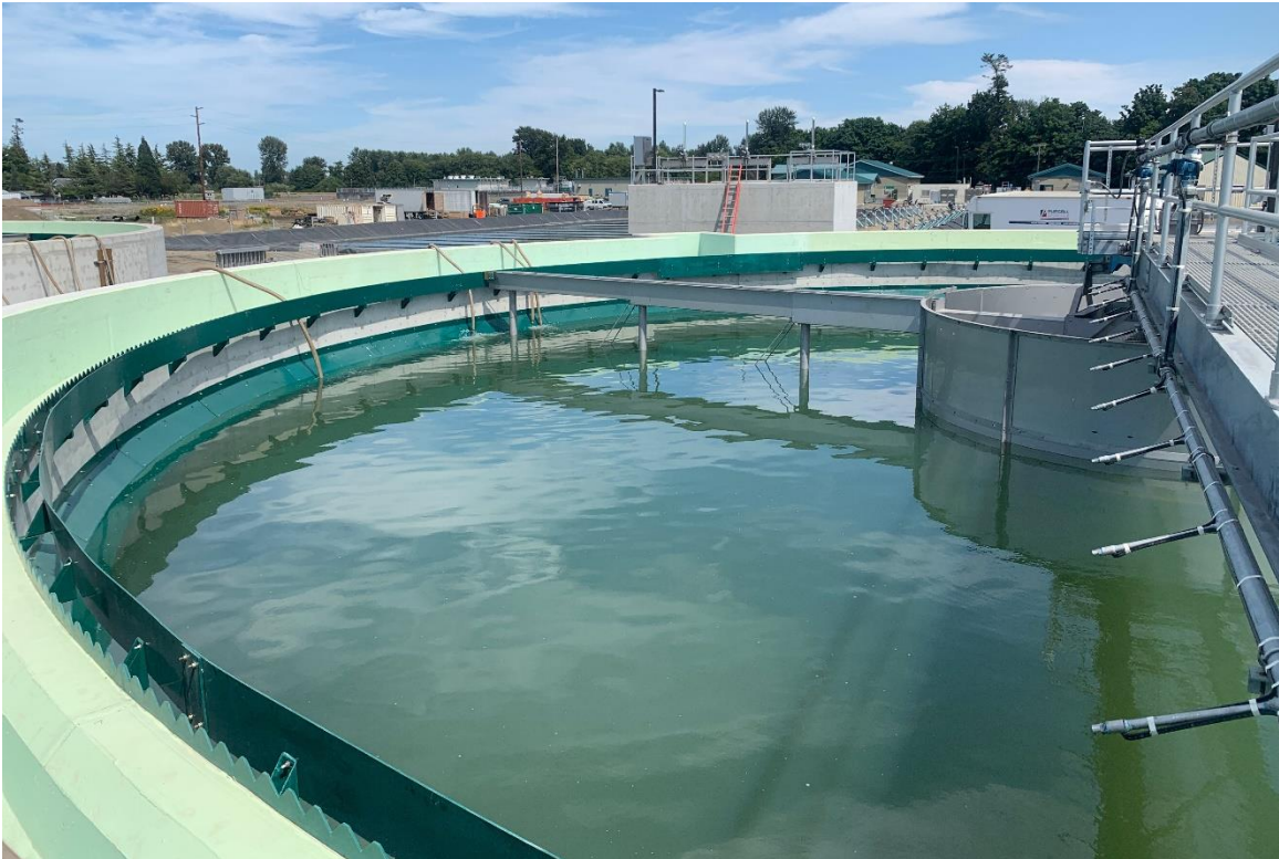
Wastewater Treatment Plant South clarifier
