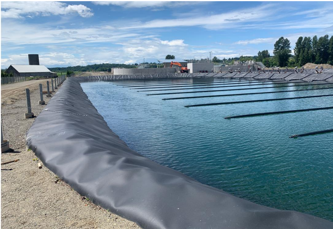
Wastewater Treatment Plant South aeration basin
