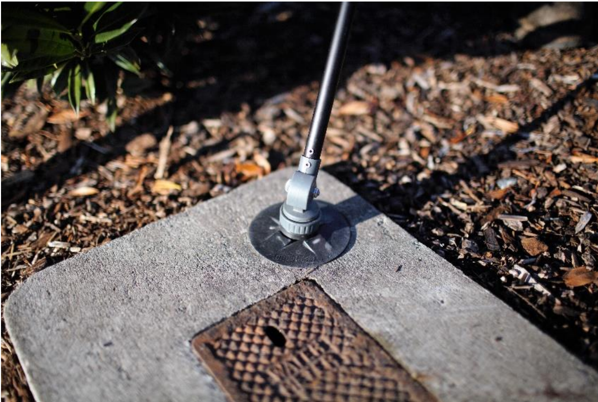
Ferndale water meter
