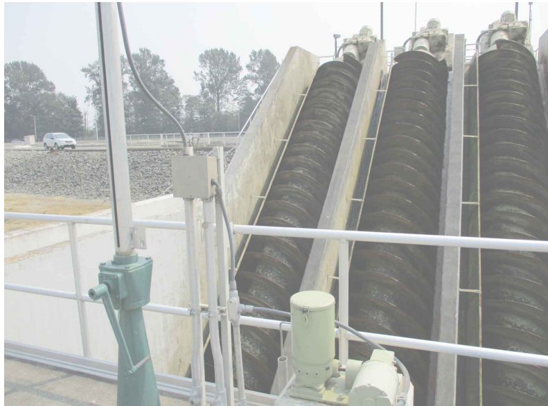
3 S2.15 TYPICAL ARCHIMEDES SCREWS NOT TO SCALE
