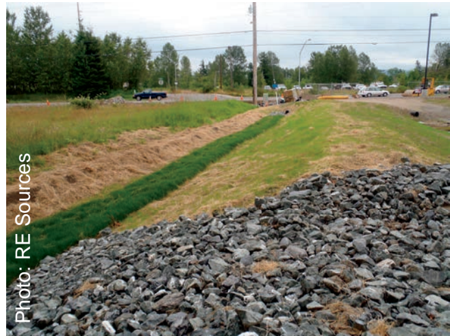
A well-maintained ditch with new vegetation layered on the bottom
