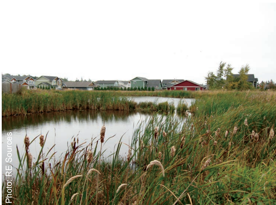
A two stage constructed stormwater pond with berm
