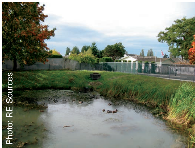
Well-trimmed vegetation makes a detention pond's outlet and fencing clearly visible.
