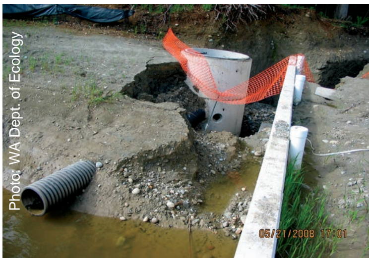
Settling, sloughing, and erosion can be signs of serious problems that lead to failure of the pond wall
