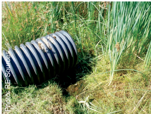
Vegetation should be cleared from around this inlet
