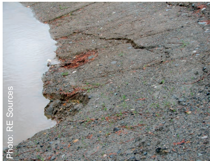
Settlement and sloughing of a pond side slope
