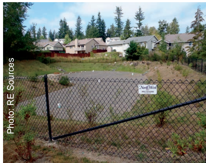
Dry pond bottom, with fencing, walls, inlet and control structure visible
