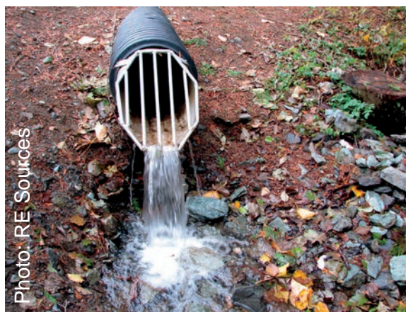
Beneath the outlet pipe is a pad of large rock, an energy dissipater , that slows fast-moving water. There may also be a dissipater below the inlet to your pond.
