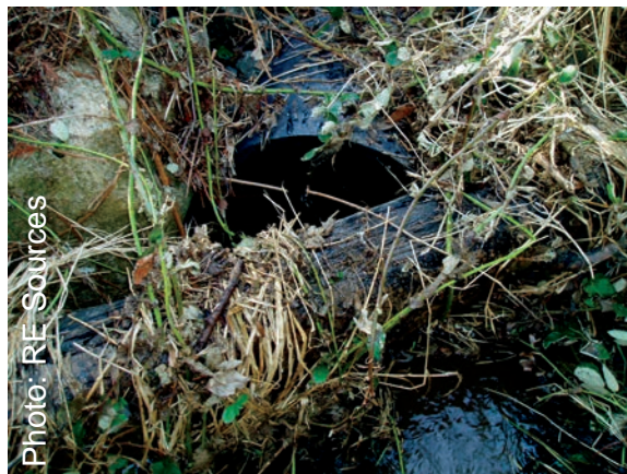
Vegetation and obstructions should be removed from clogged inlets
