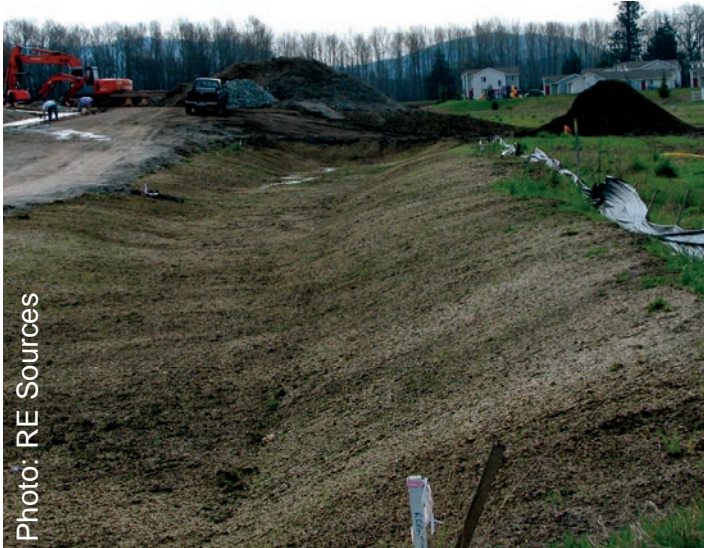
A bioswale under construction
