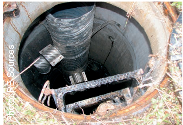
Control structure inside a Type 2 catch basin
