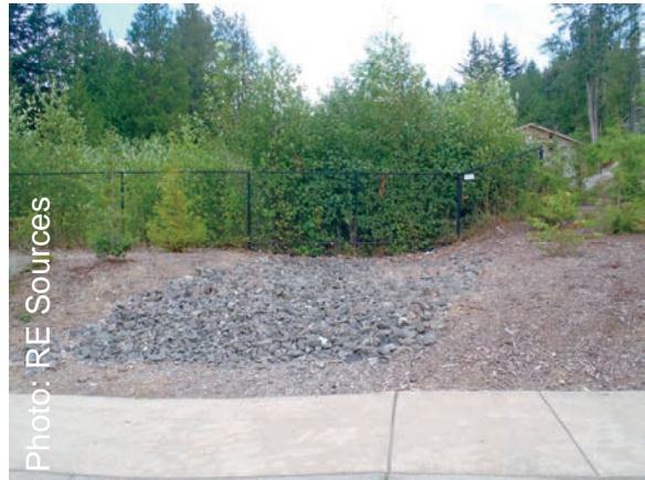
Water only passes over the spillway when the pond fills up.
