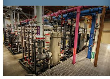
We are pleased to say this new Reverse Osmosis system has reduced the hardness levels. It has also drastically reduced our use of chlorine required to treat the water to ensure quality and safety.
