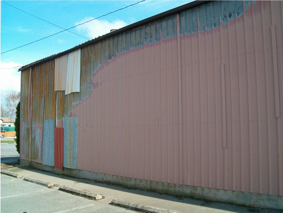
Fire Damage at Northwest Corner
