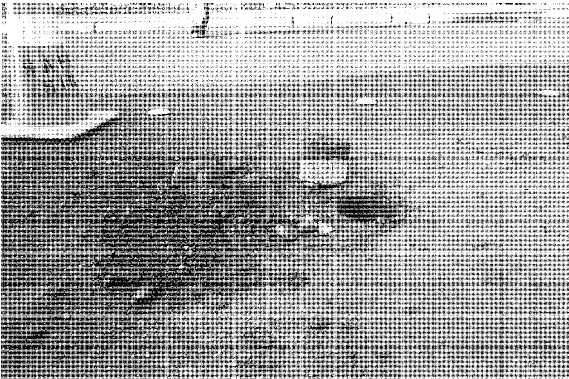
Looking West on Church Rd. – Location 12 (Date Incorrect)
