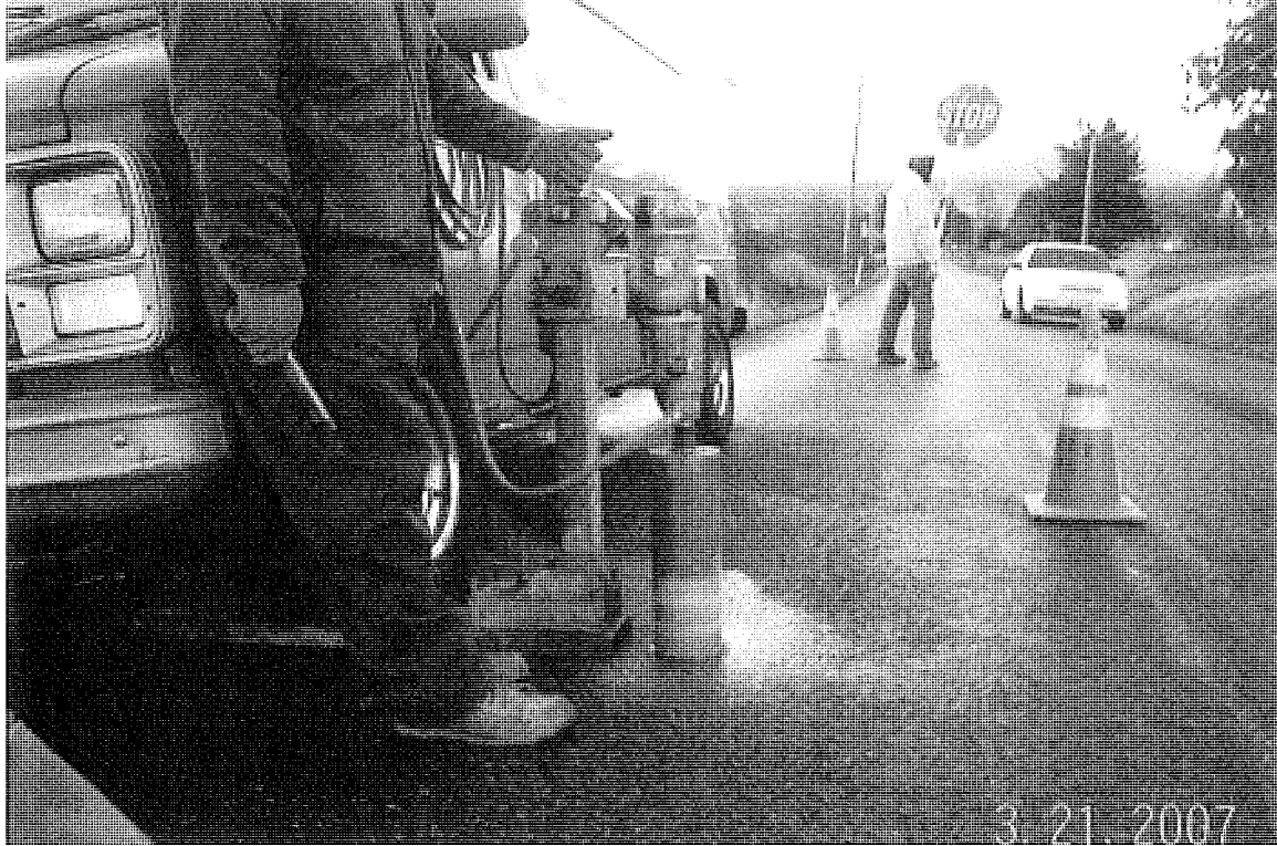
Looking South on Church Rd.- Location 9 (Date Incorrect)
