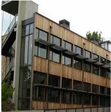
Utilize natural lighting by having large windows and skylights; also known as daylighting. Orient the building based on the rotation of the suns path to maximize natural light to reduce the use of artificial light.
