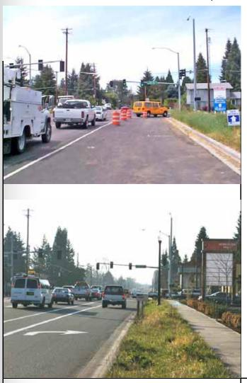
Before and after photographs of road improvements showing the construction of a right-hand turn lane, bicycle lane, curb, gutter and sidewalk Depending on the intensity of proposed uses, traffic mitigation shall be completed prior to occupancy.
