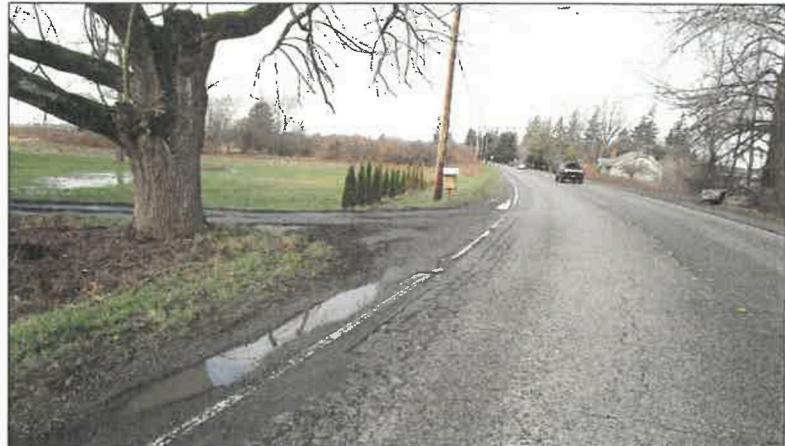
This project consists of widening of the roadway to City standard, including 5' wide shoulders, new sidewalks, crosswalks, streetlights, and bus pullouts. Stormwater improvements will protect Tenmile Creek/Barrett Lake.
