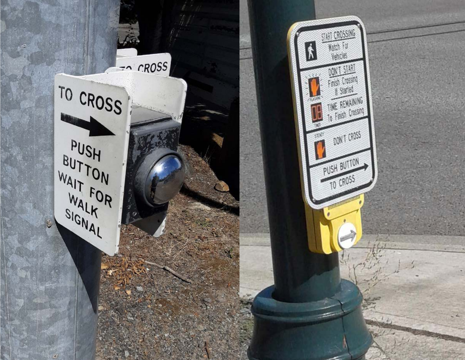
Figure 2-17 “H-style” (left) and APS-style (right) pedestrian pushbutton
