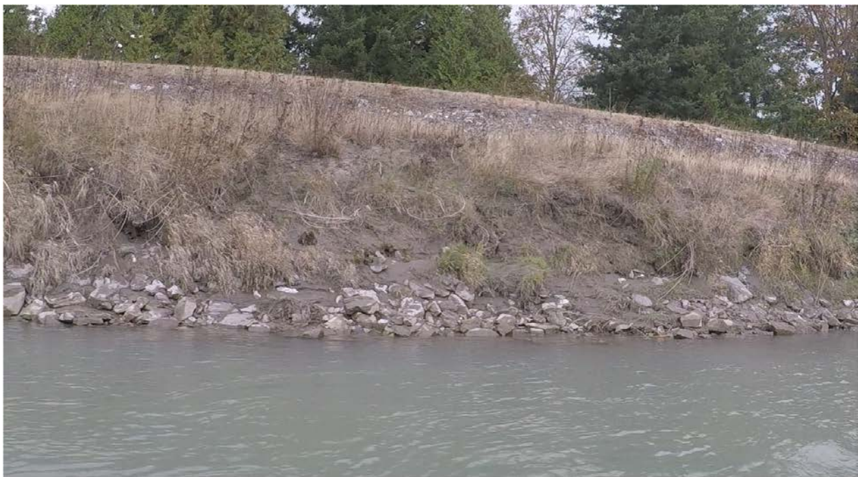
Figure 10 Station 69+00, location of significant sloughing and armor loss
