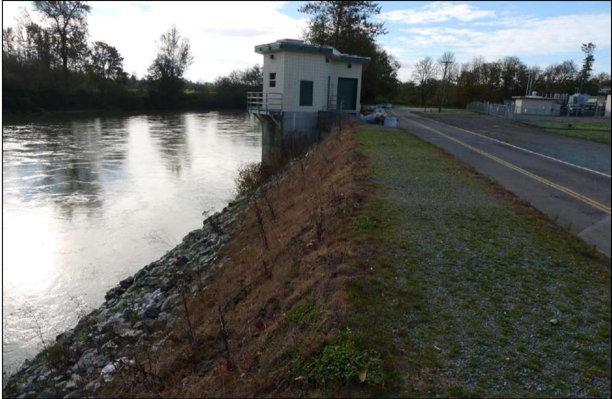
Photo 4. Overview of riprap along the levee. View is south.
