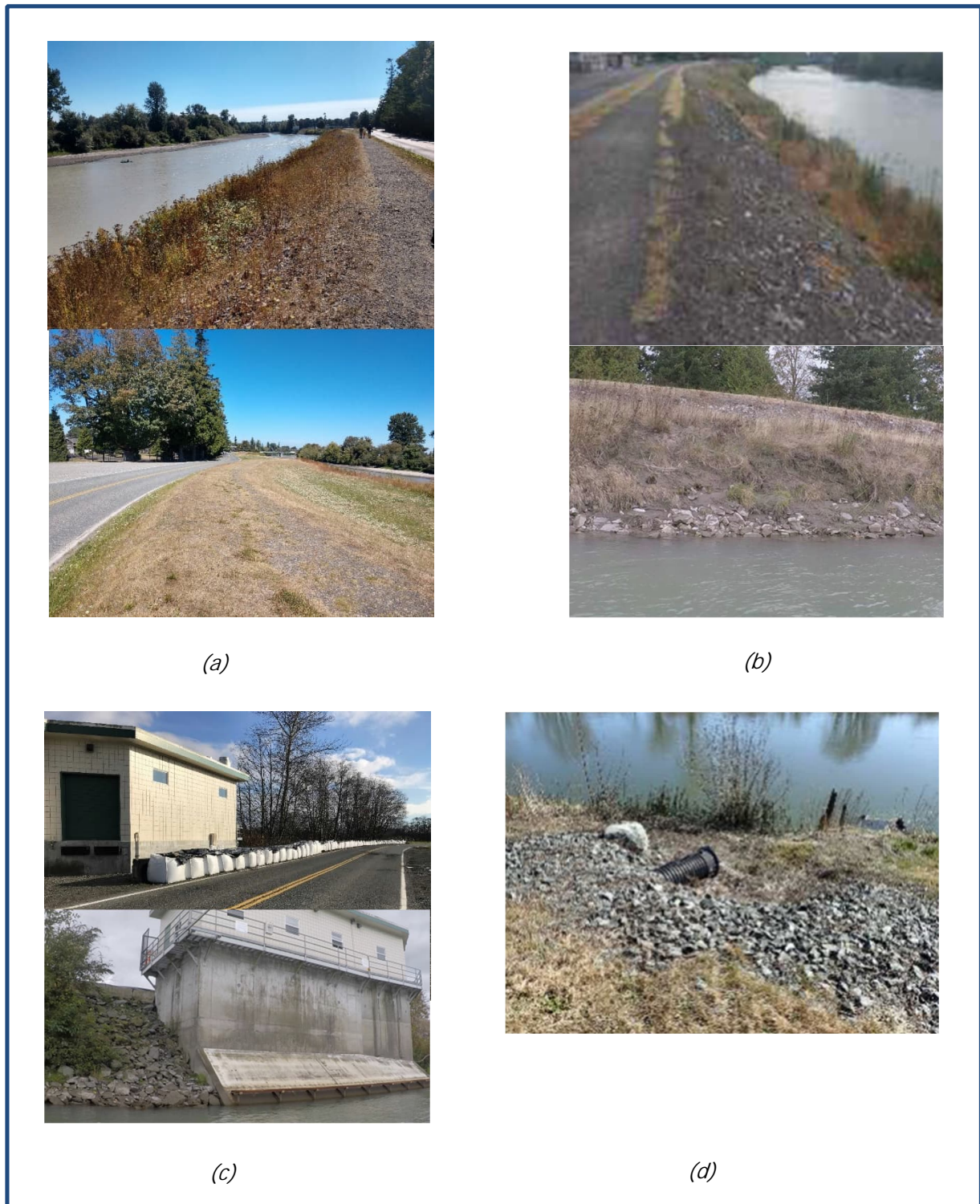
Figure 5: Recent inspection and Site Visit Photos of the Ferndale Levee; (a) Levee and trail across from Pioneer Park – facing south (top) and north (bottom) – narrow crown (b) Erosion and sloughing areas across from Pioneer Park – viewed from land (top) and water (bottom); (c) PUD No. 1 intake structure and super sack closure structure – viewed from road (top) and water (bottom); (d) Culvert penetration across from Star Park
