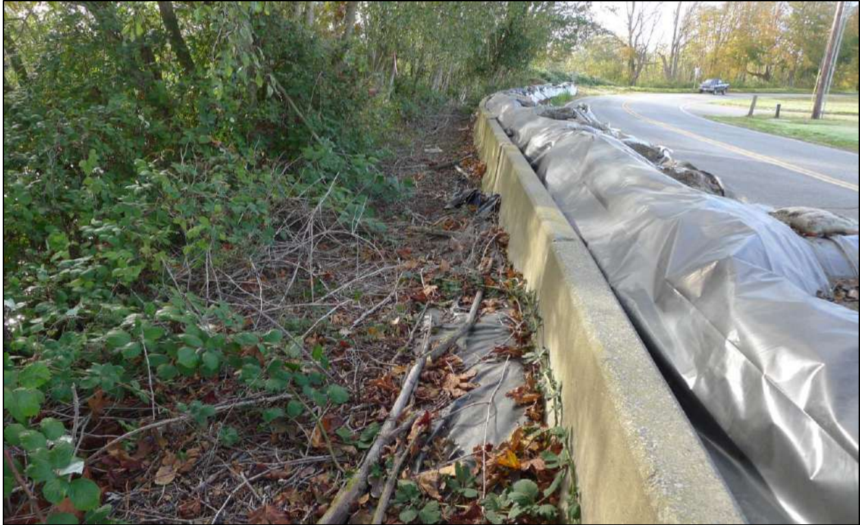
Photo 6. Concrete and sandbags installed along the levee and Ferndale Rd. view is south.
