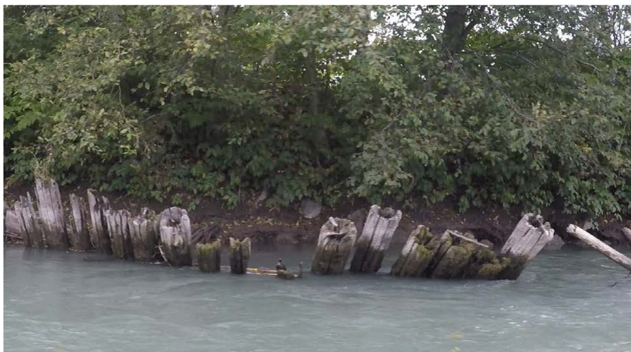
Figure 12 Ferndale WTP Sta. 26+00, location of significant armor loss, steep banks, and wood piling degradation
