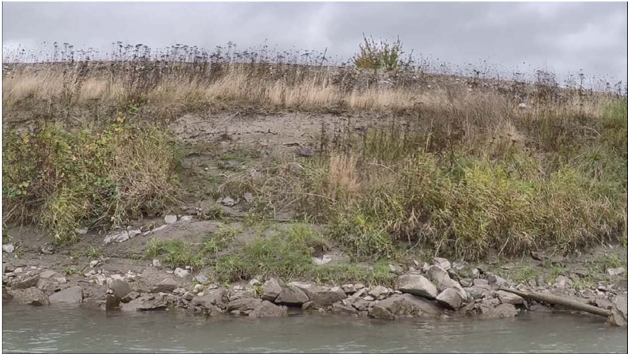
Figure 9 Station 75+50, location of significant sloughing and armor loss
