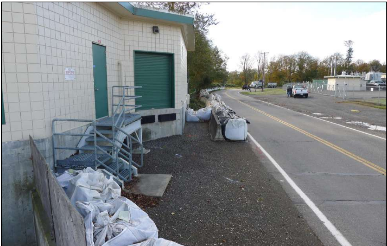
Photo 5. Sandbags, concrete, and eco-blocks installed along the levee. View is south.
