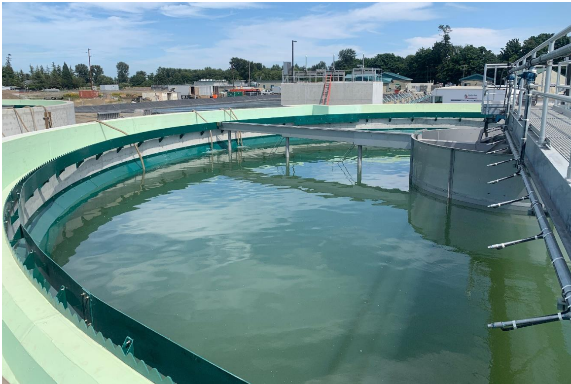
Wastewater Treatment Plant South clarifier
