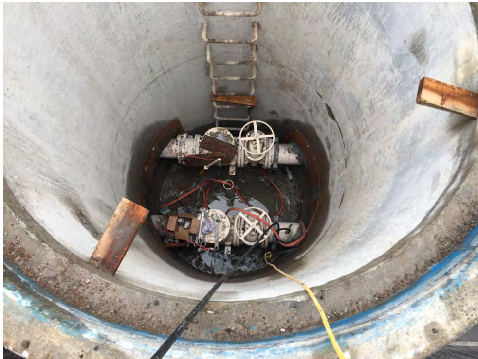
PS#4 Discharge Valve Vault
