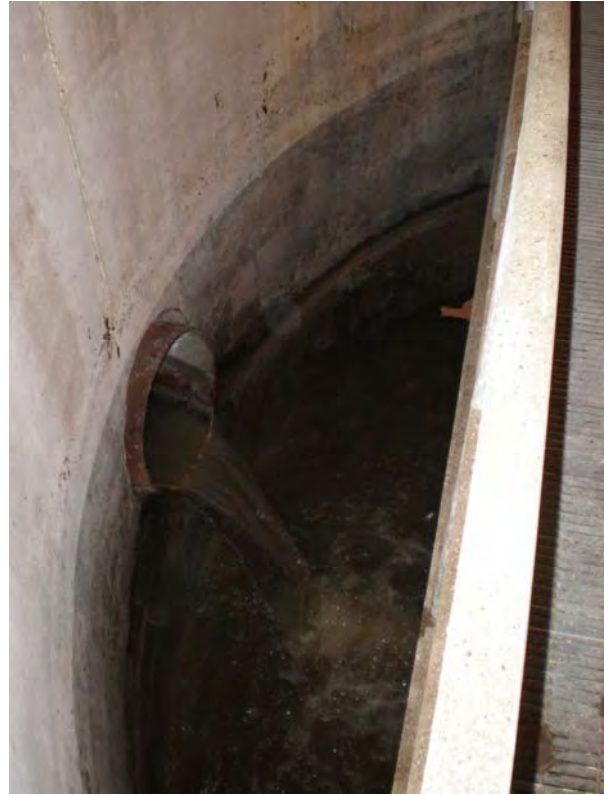
PS #2 Wetwell Influent Pipe
