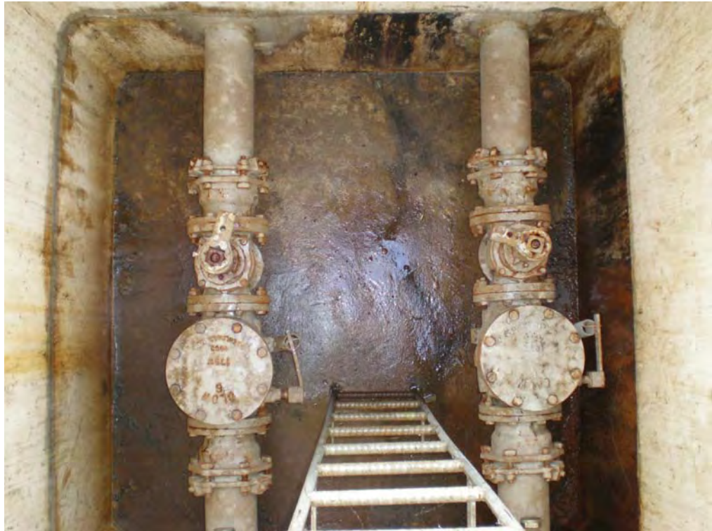
PS#16 Discharge Valve Vault
