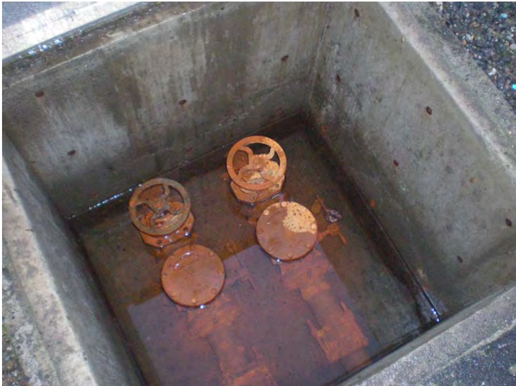
PS#18 Discharge Valve Vault
