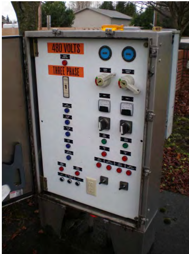
PS#15 Control Panel
