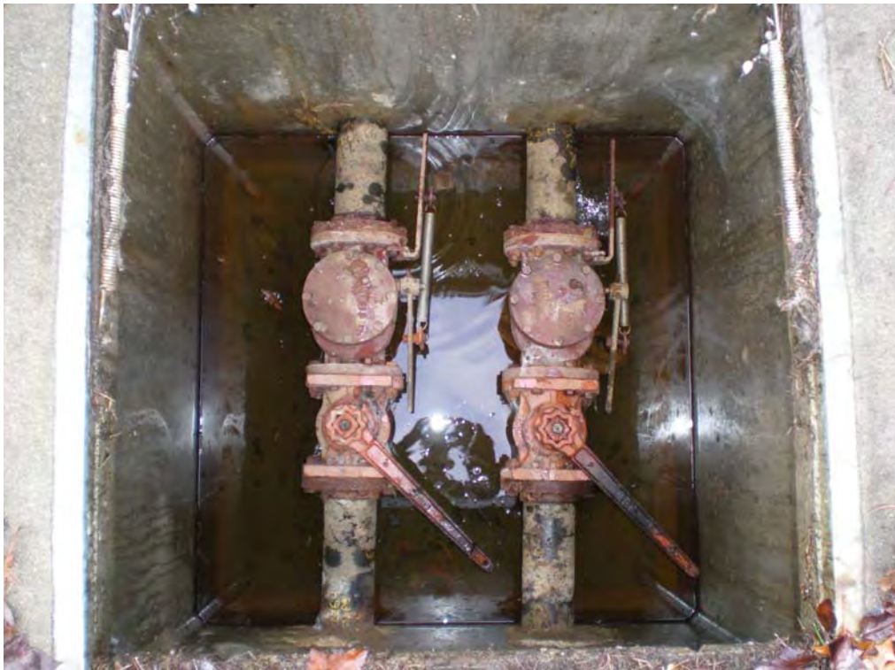
PS#6 Discharge Valve Vault
