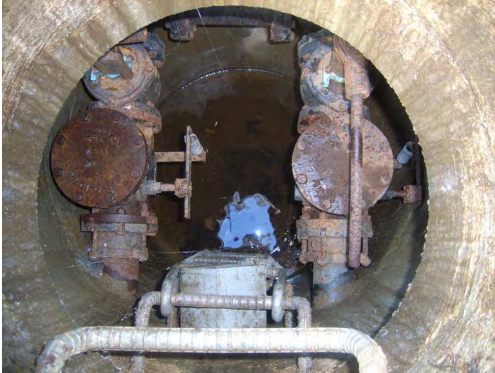
PS#5 Discharge Valve Vault
