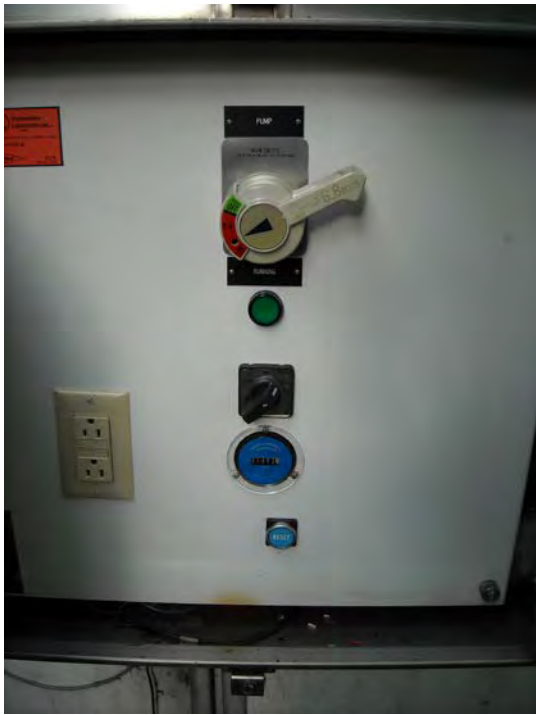
PS#12 Control Panel
