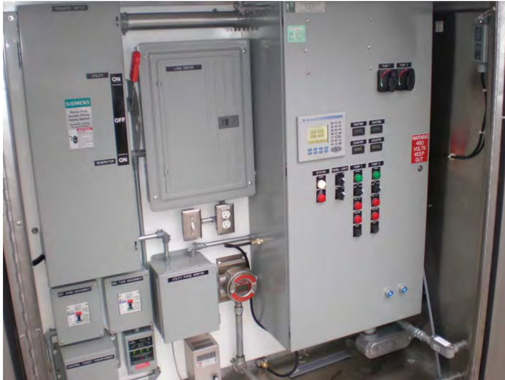
PS#22 Control Panel
