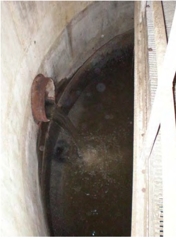
PS#3 Wetwell Influent Pipe
