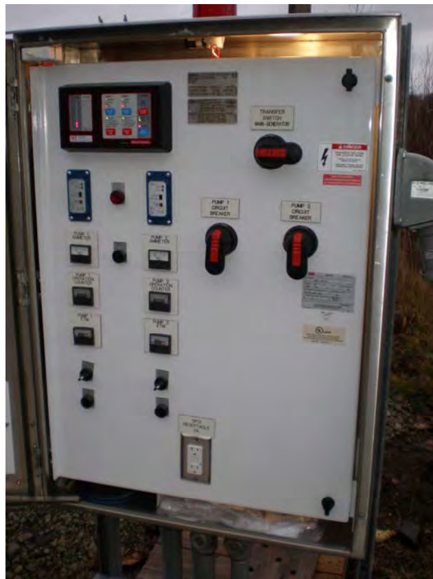
PS#19 Control Panel
