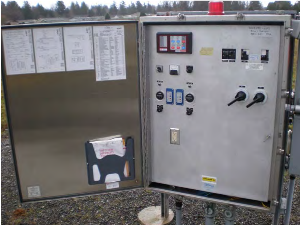
PS#9 Control Panel
