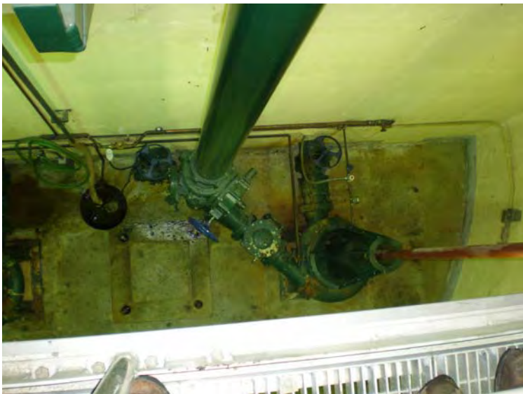
PS#3 Dry Well Pumps
