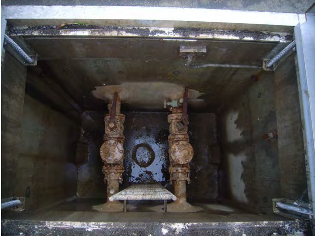
PS#17 Discharge Valve Vault
