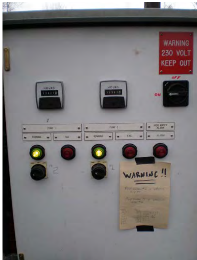
PS#11 Control Panel
