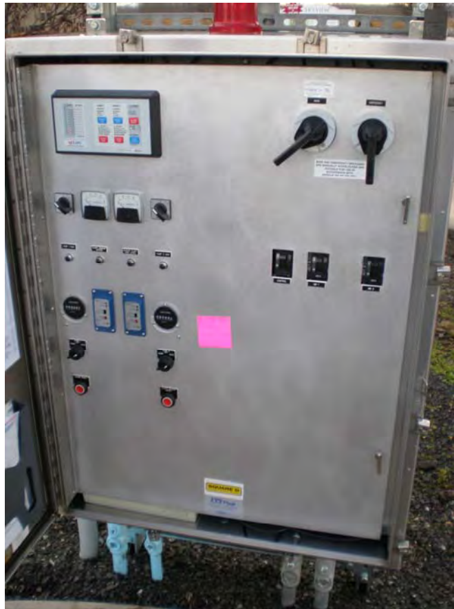
PS#20 Control Panel
