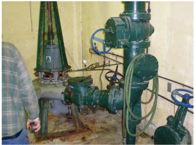
PS#2 Dry Well Pumps
