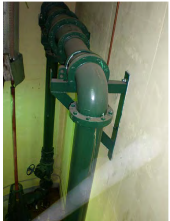
PS#3 Discharge Line
