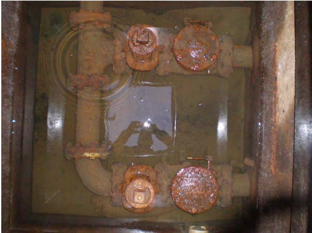
PS#10 Discharge Valve Vault
